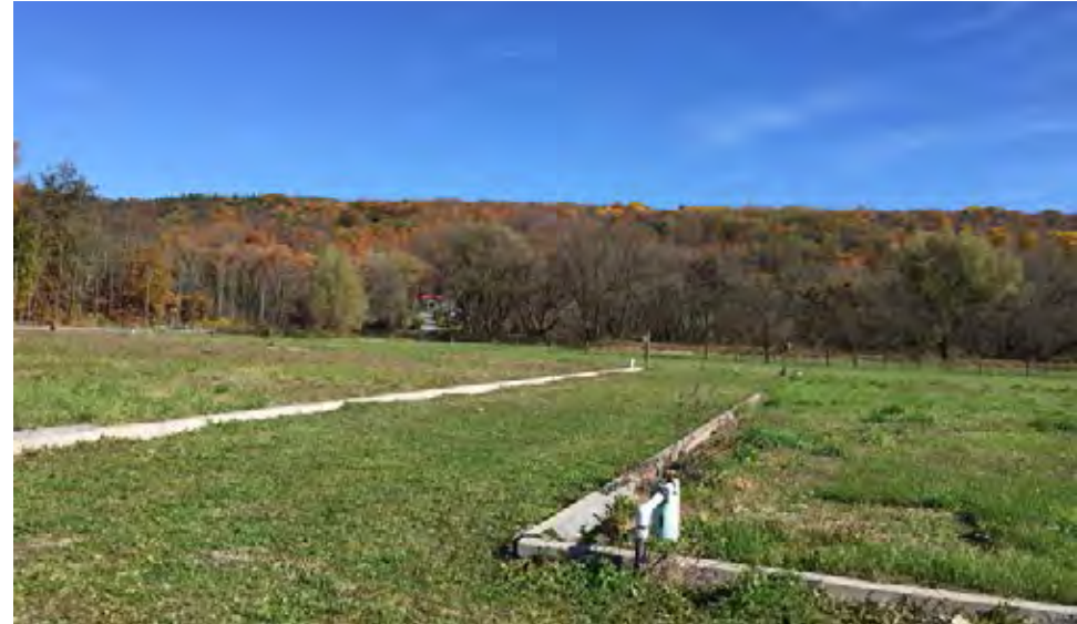
The Town has four leach fields for wastewater management located along Kellogg Road west of N Main Street (Route 15A).
